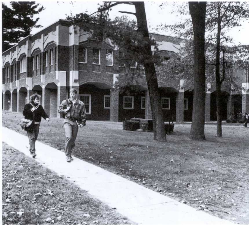
Knight Annex has become Malloy Hall, a two-story building containing classroom and faculty offices. It was named for James B. Malloy '51, whose generosity made the building possible.
